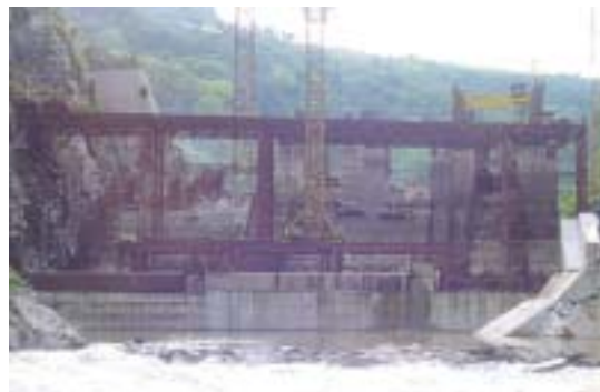
Huge projects require large amounts of timber for adequate housing infrastructure
